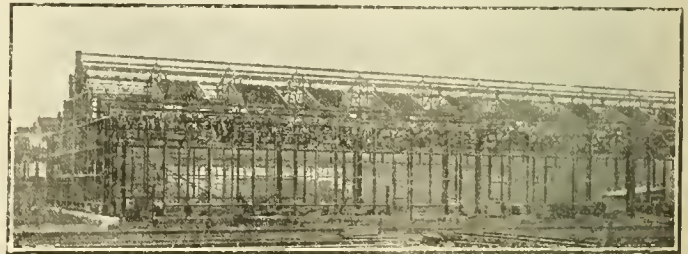
CONSTRUCTION VIEW OF THE PASSENGER CAR ERECTING SHOP. (FROM SOUTHEAST CORNER.)
